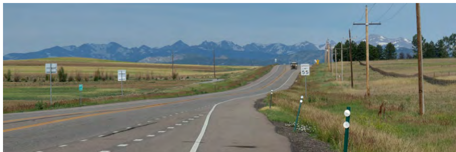
CO 52 (MP 3) looking west along corridor
