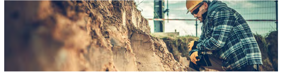
Roadway improvement projects must consider sensitive archaeological and paleontological resources prior to development
